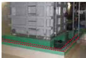
Drainage dikes *Red frame indicates a drainage dike. Installation of drainage dikes to prevent leakage of fluids and underground seepage when wastewater is spilled from tanks.
