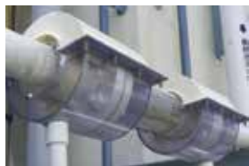
Double joints in piping Installation of double joints in piping to enable checking for leakage of fluids.
